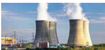
Power generation & distribution
